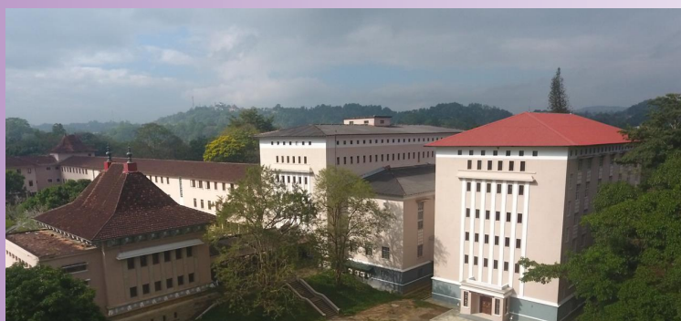
Library Building University of Peradeniya with new extension (Photo by Author)
